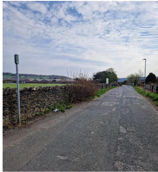
Photo 1: Application route commences at the south west corner of the Cricket Ground, east of No. 43 Mean Lane (Point B on the Application Map in Figure 2). First 150m of Application route is metalled with four street light columns and the width is predominantly 6m but varies between 9m and 4m and is accessed.
